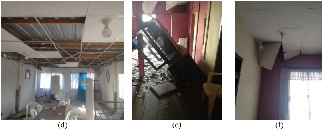
Figure 14. Damage to non-structural components and building contents.
