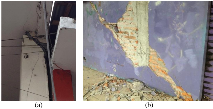
Figure 10. Brittle failures due to pounding (a) and interaction between RC frame and infill wall (b).
