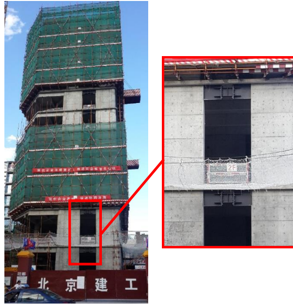
Figure 16. Illustration of Sancai Building adopting a HCW system with RSCBs.
