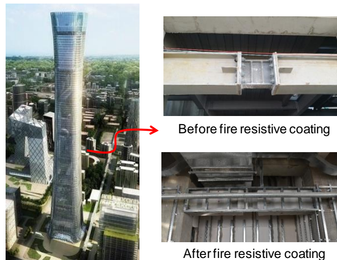
Figure 19. Illustration of China Zun Tower (Beijing Z15 Tower) adopting RSCBs.
